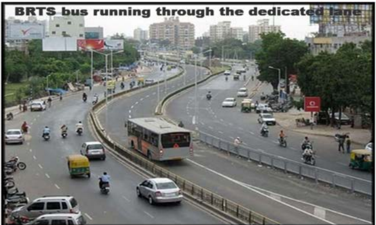
Figure 7: BRTS Dedicated Lanes
